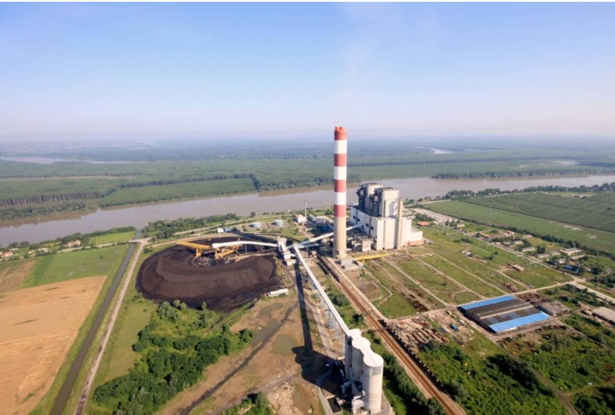
TPP Nikola Tesla TENT B, EPS, Power Utility Serbia
