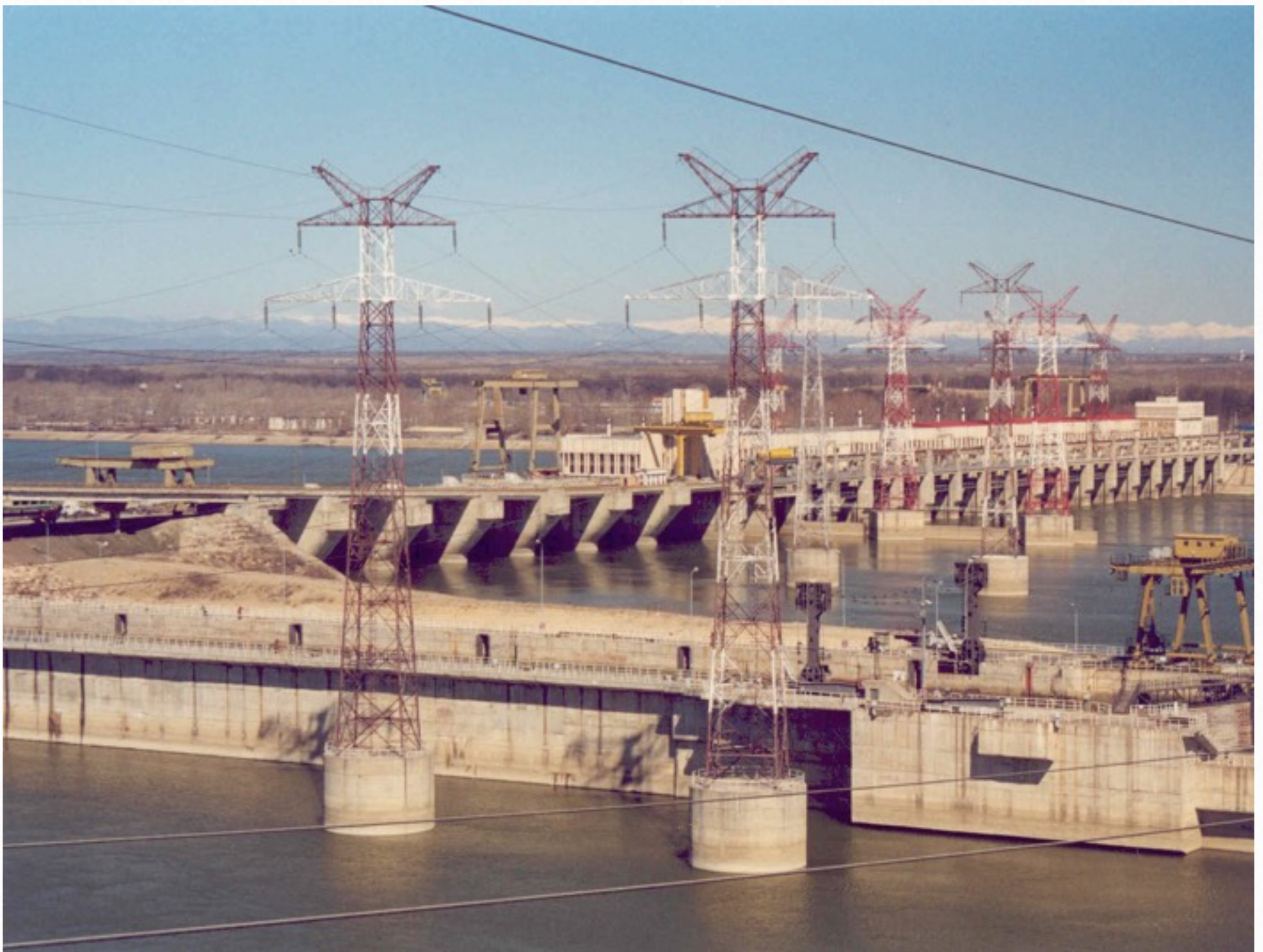
HPP Djerdap, EPS, Power utility
